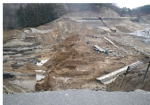
Fig. 2 被災直後の藤沼ダム Fujinuma dam immediately after collapse
